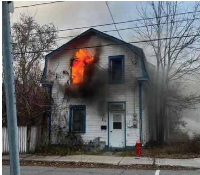
Old Aylmer home located at 81 rue du Couvent with flames blazing from the second-floor window, taken by a resident passing by the home (SD)
