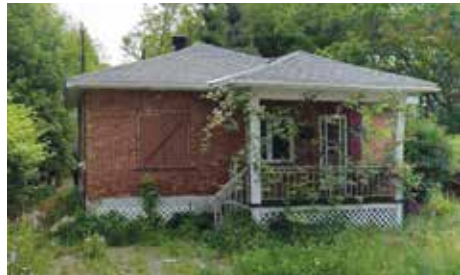
The current building at 30, rue Bancroft slated for demolition
