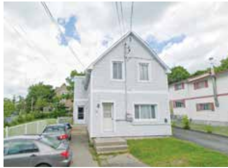
The two-unit house at 17, rue du Centre slated for demolition
