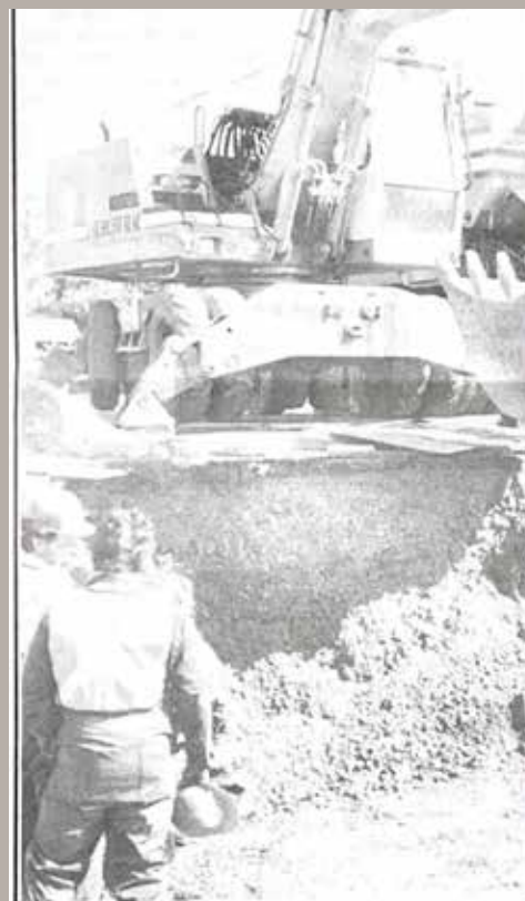
ANOTHER SIGN OF SPRING Workmen study the impact a digger has on city streets. Another slowdown for the hapless motorist Rick Antonishin photo
